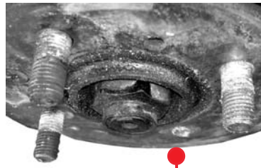
Sheared off lug bolt
