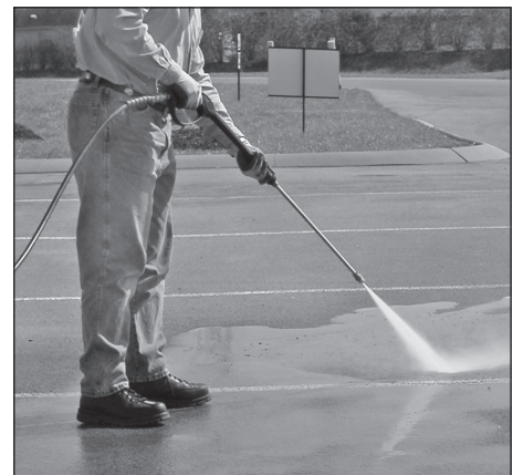
Figure 13 - Optimum angle to cleaning surface
