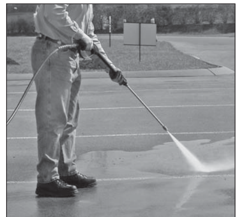
Figure 20 - Optimum angle to cleaning surface
