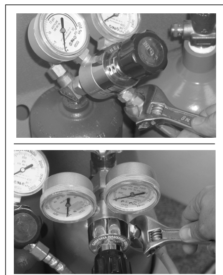
Figure 3 - Acetylene Connection (top) and Oxygen Connection (bottom)
