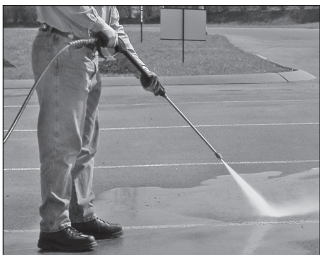
Figure 11 - Optimum angle to cleaning surface
