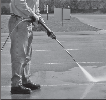
Figure 11 - Optimum angle to cleaning surface
