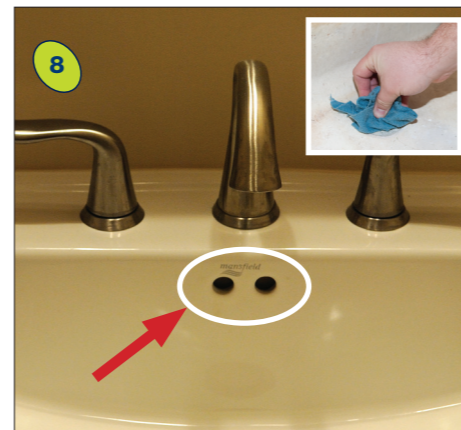
Cover any overflow opening in the sink with a wet rag or duct tape. If using a double sink, put a rag in the other drain opening.
