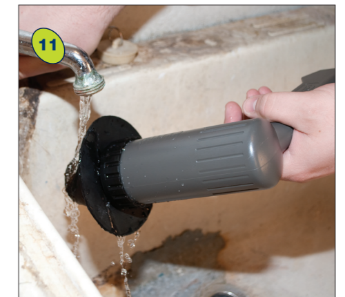
After blockage is removed, flush drain using plenty of water to carry the blockage material well away from water lines. Check sink traps and, if necessary, tighten up leaking joints. Wash off drain cleaner with clean water.
