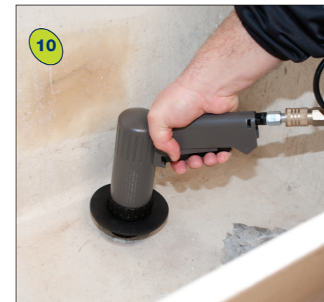
If blockage is not removed, repeat step 9. Add more water if necessary and increase air pressure slightly. Do not exceed 50 psi. Wait several seconds between air pulses to avoid pressurizing the drain system and damaging the pipes.
