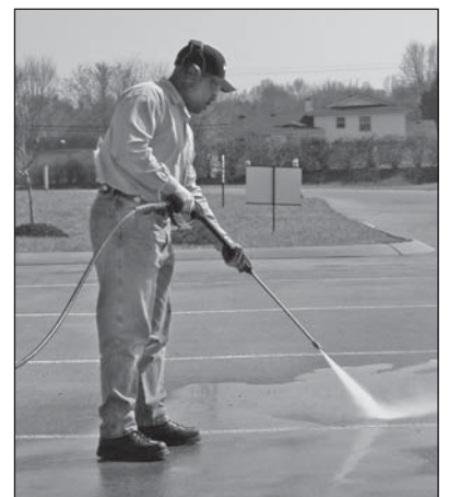
Figure 15 - Optimum angle to cleaning surface
