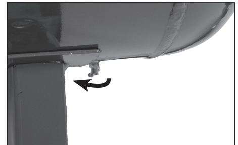
Figure 16 - Manual Tank Drain
