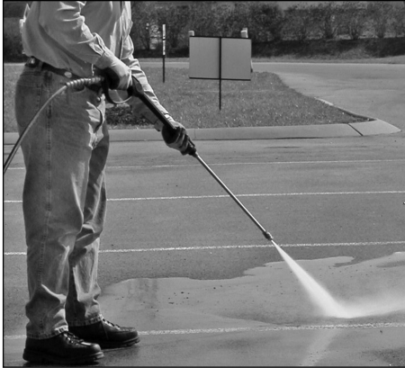
Figure 12 - Optimum angle to cleaning surface
