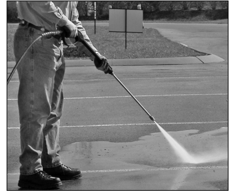
Figure 14 - Optimum angle to cleaning surface
