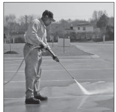
Figure 16 - Optimum angle to cleaning surface
