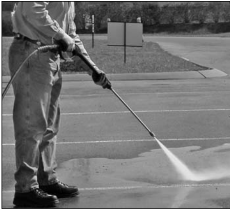
Figure 12 - Optimum angle to cleaning surface
