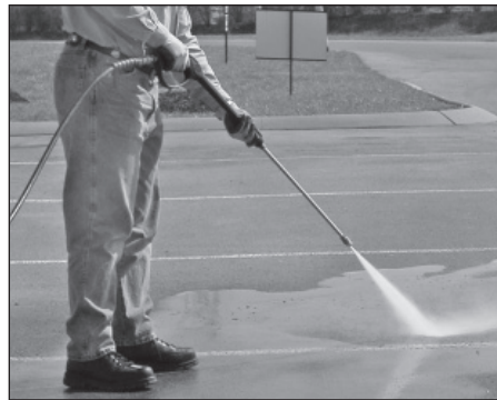
Figure 14 - Optimum angle to cleaning surface
